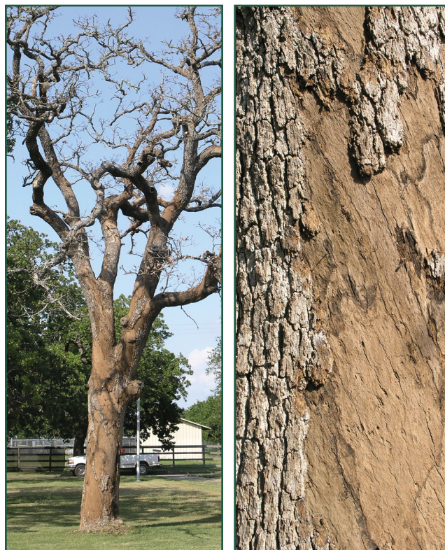
Figure 1. Exposed cankers of Biscogniauxia atropunctatum on a post oak after the tree dies and the bark sheds. Source: David N. Appel
